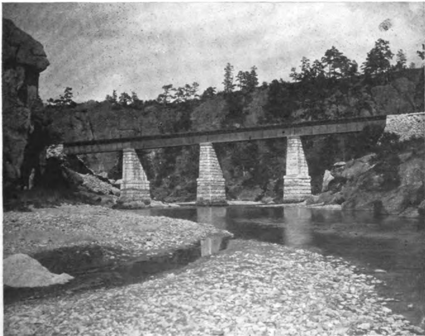
Steel Bridge across Guerrero River.
